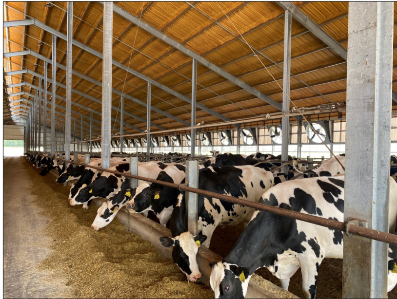
Figure 1. WILRA Farms' new barn with an all-seasons hybrid ventilation system.
